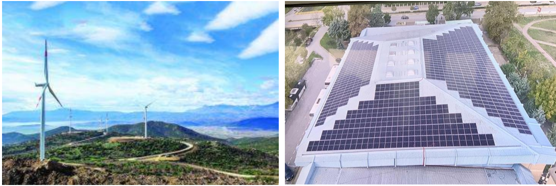
Figure 3 Renewable wind and solar installations in South-East region
